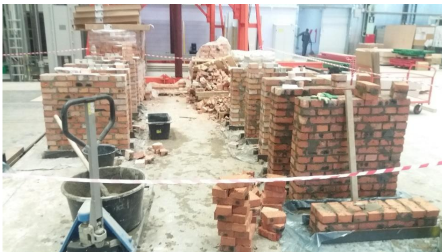
Figure 1 – Samples of brickwork
