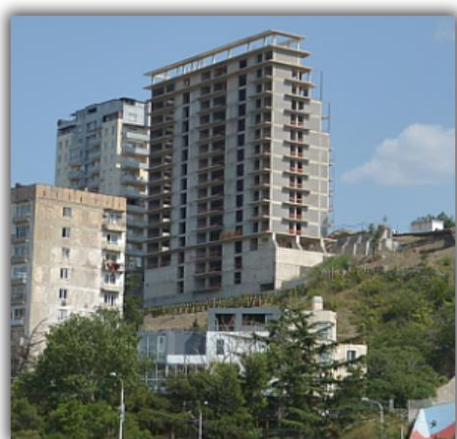
Fig. 1 The multistory building on the slope
